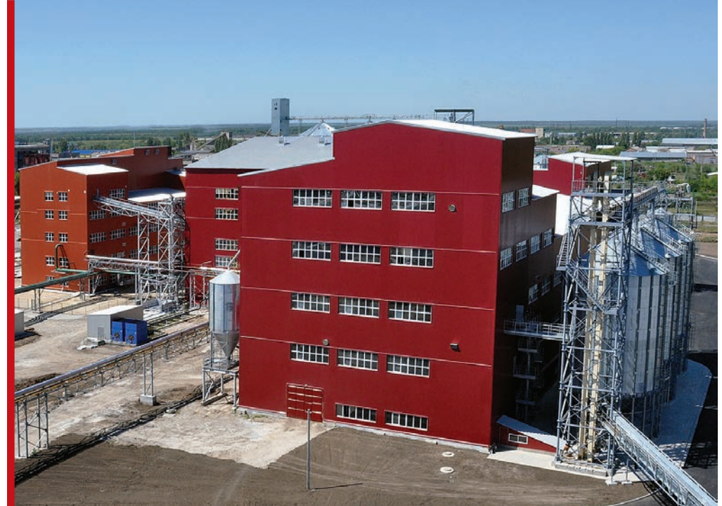
05. | COMPLETED PLANT JULY 2012
