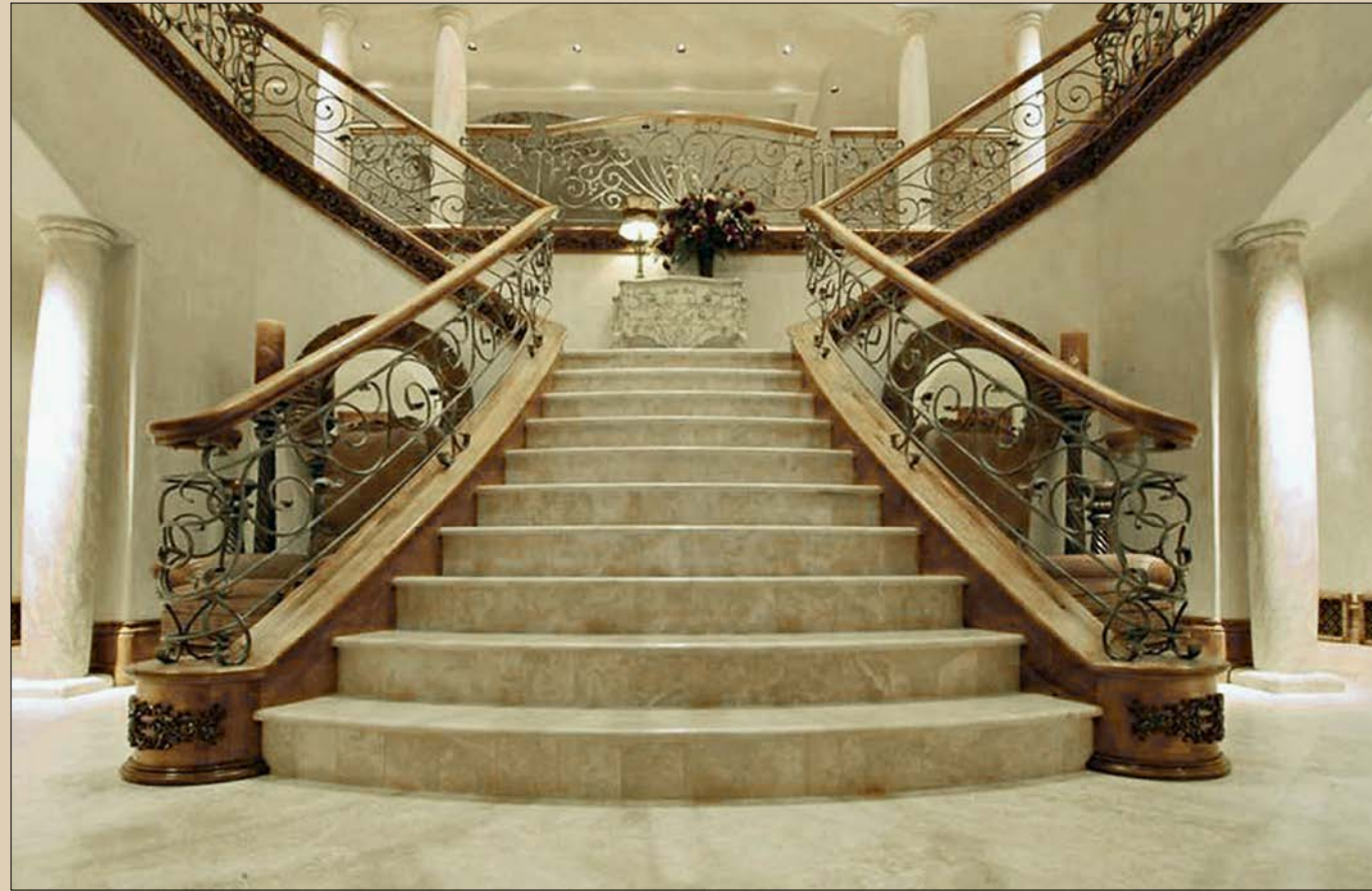
Stairs (marble with art forging)
