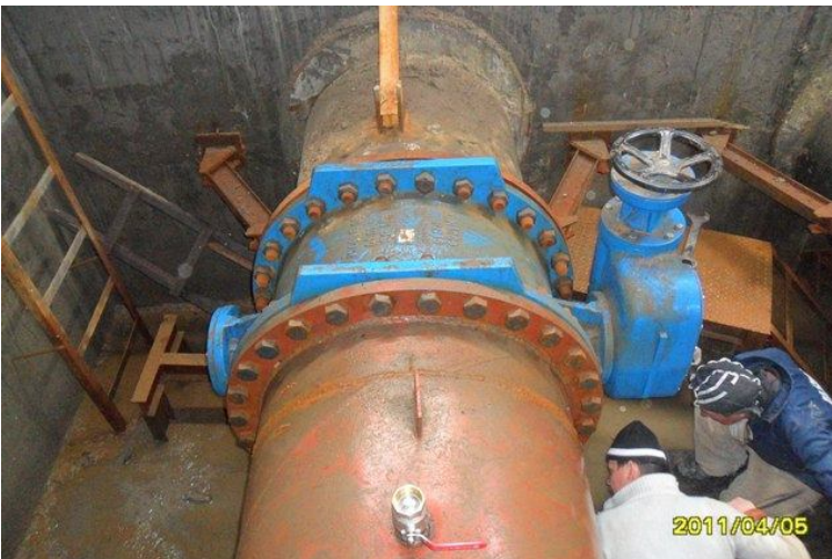
Manually adjustable flow control valves, above and under
